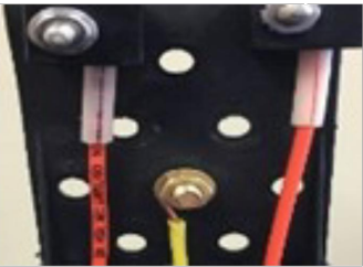
Install TRACE-SAFE and ground wire using TS-MPC no-strip connectors
